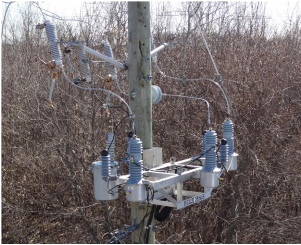
Auto-grounding system with series-connected fuse
