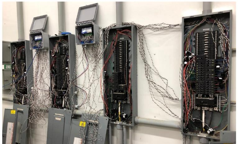
Data loggers with electric current sensors connected and installed in Farm B's circuit panel boxes.
