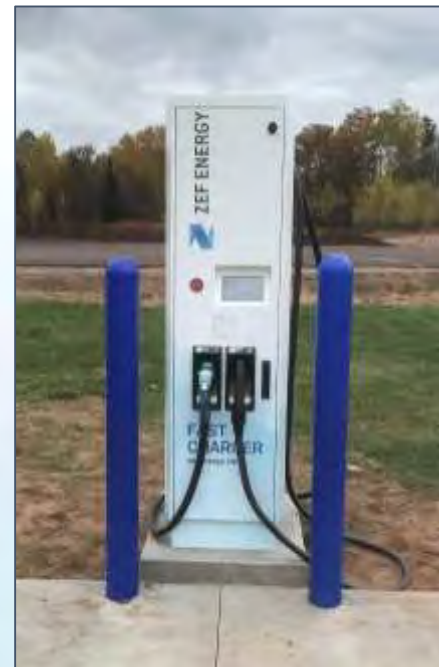
ZEF DC 50kW Fast Charger Cost range: $60k - $150k installed (range for 50kW-150kW chargers)
