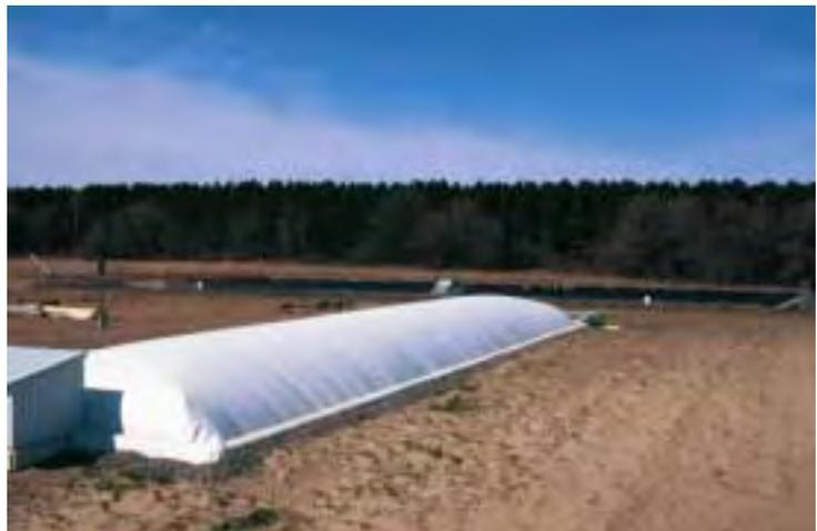
**Anaerobic plug-flow digester. Haubenschild Farms, Inc.**
