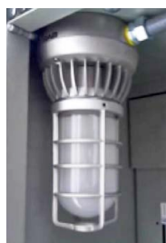
Figure 3. LED jelly jar with heat-dissipating design.
